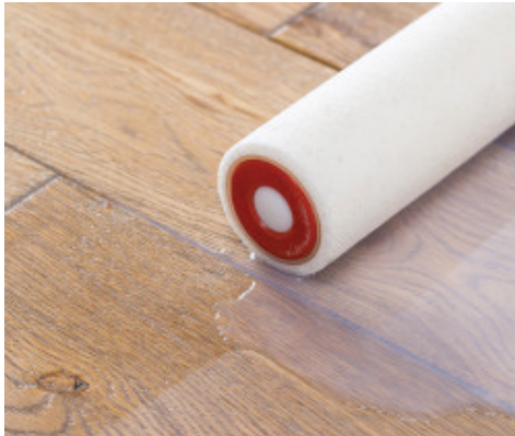
After sanding application of Ultracoat two-component, water-based varnish
