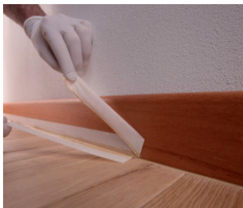
Removing the protective paper tape
