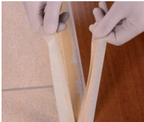
Removing the protective paper tape
