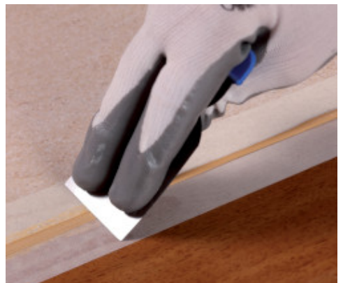
Finishing off the surface
