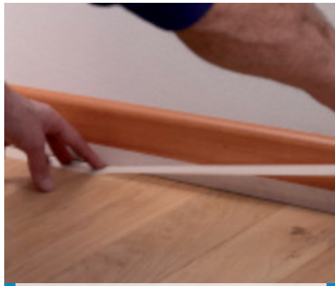
Protective preparation of the sealing of the joint
