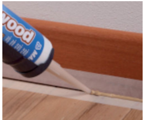
Filling the joint
