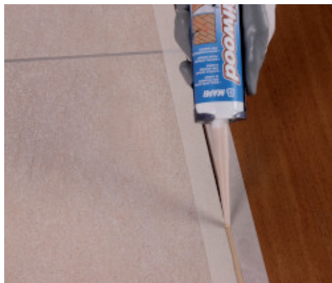
Filling the joint
