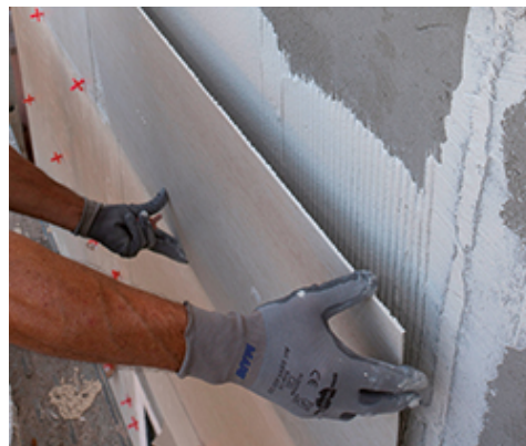
Applying a thin porcelain tile on external façade
