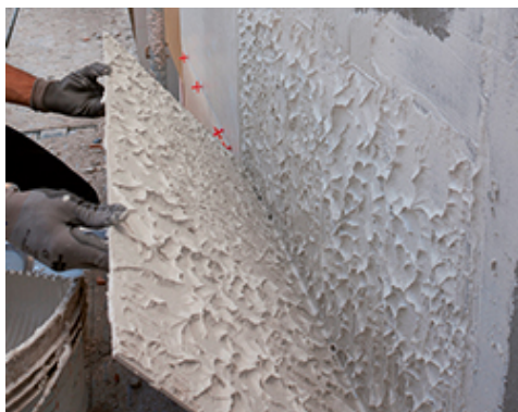
Checking the back face of the tile if it is completely buttered when laying on an external façade
