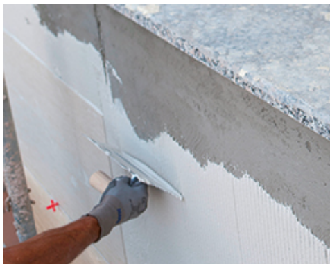
Laying on an external façade: application of adhesive on the substrate
