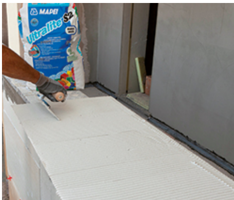
Spreading the adhesive on the back face of the tile
